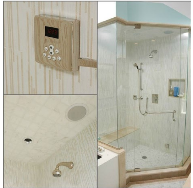
Top Left: Mr. Steam steam bath controls. Bottom Left: Ceiling installed steam misters. Right: Shower with steam bath, wall mounted and hand held showerheads, grab bar, bench seat and wall niche.
