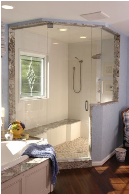
Custom walk-in shower with granite accents and river rock tile.
