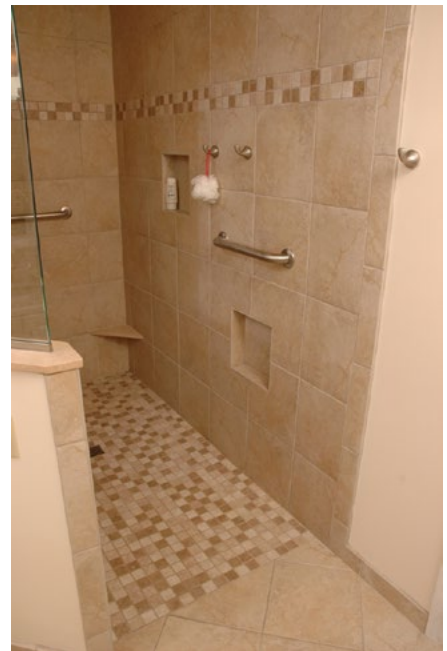
Walk-in shower with a level threshold and no door.
